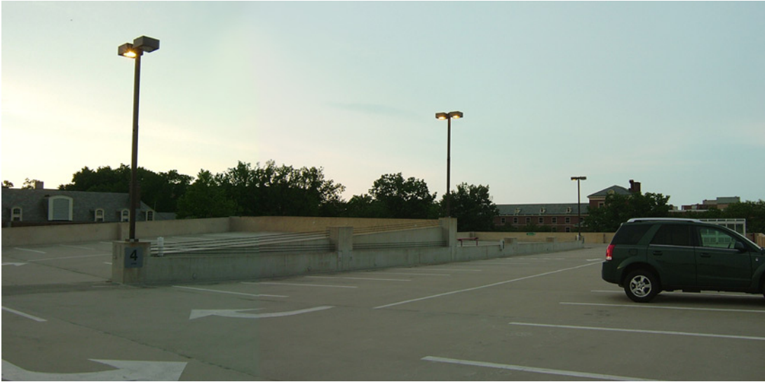
Fig. 9 A picture of the top level of the parking garage on which the tests described in this paper were performed. This picture was taken from a location in the lower left corner of Figs. 10–12 and 17.
